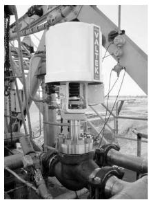
This cryogenic Mark One is used for aerospace testing as an O2 vent.
